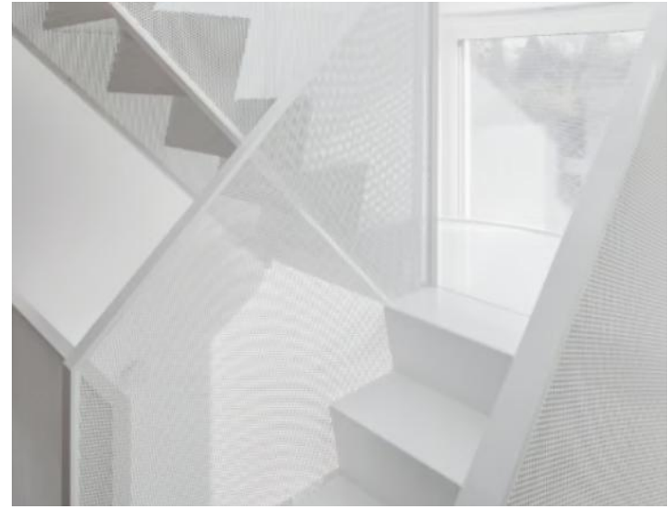
R5 T8 perforated sheet stainless steel, 1.50x1500x3000mm
